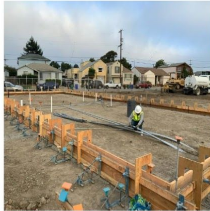
Running the utility lines
