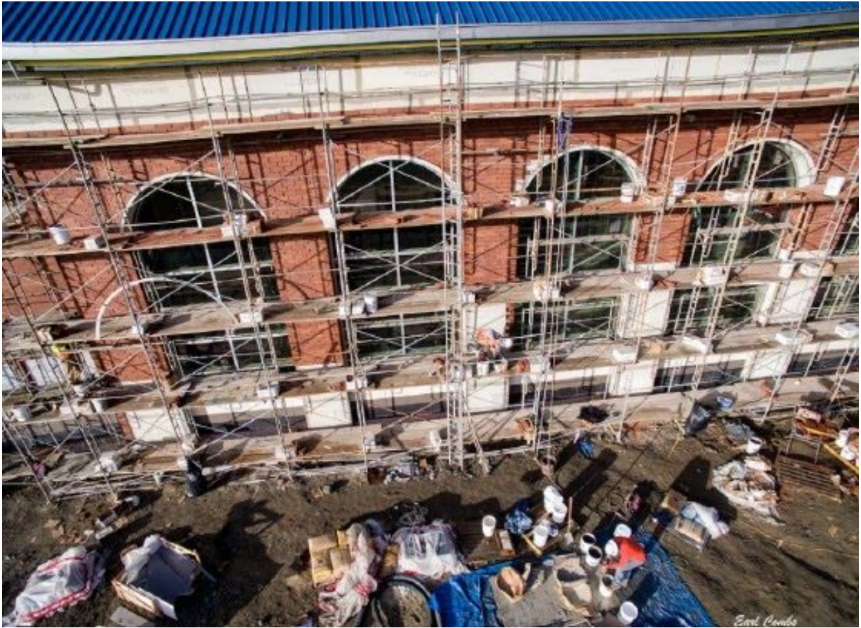
Pinole Valley High School - window installation
