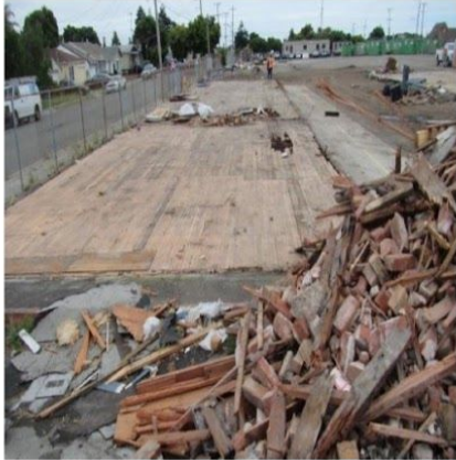
Demolition and clearing site
