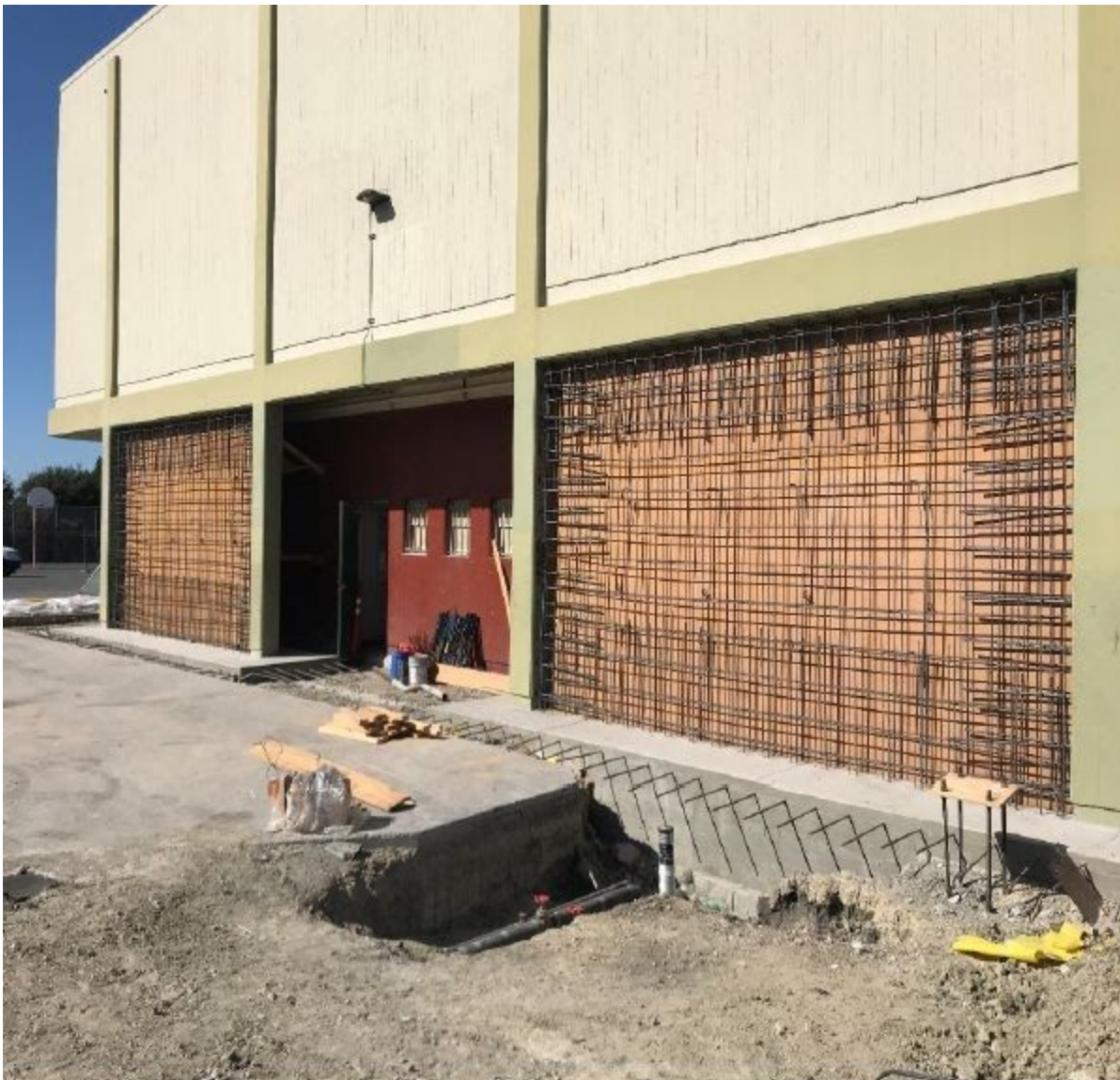
Juan Crespi Elementary school - seismic upgrade to existing two story concrete gymnasium
