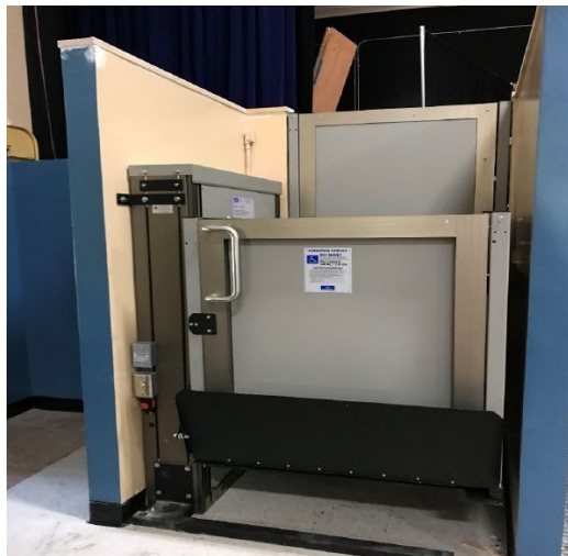
Fairmont ES - wheelchair lift to stage
