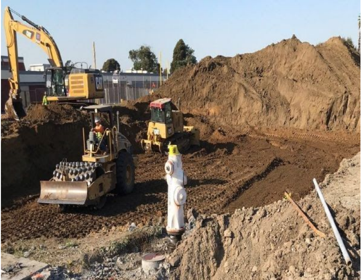
Richmond High School - Construction of a single story gymnasium
