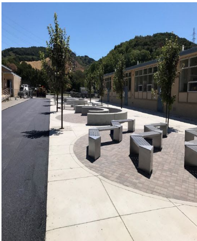
Olinda Elementary School - repair tripping hazard due to tree roots lifting concrete
