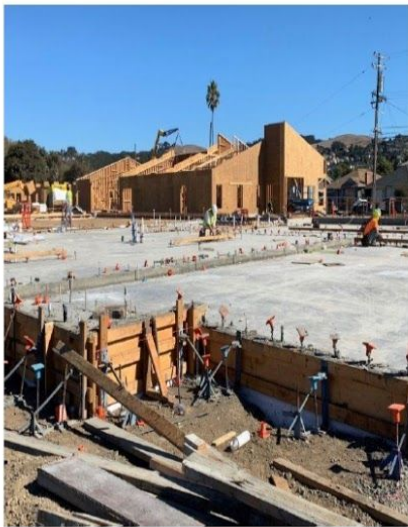
Cement slab work
